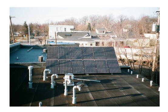
With the panels being a slightly different size, we had to re-calculate the lengths of the UniStrut members needed to build the rack for City Hall. These calculations are finished and that material will be ordered shortly.
