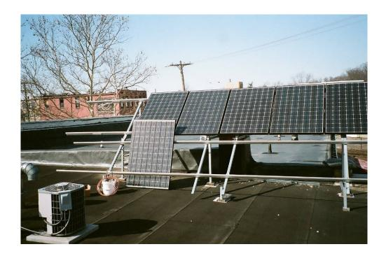
This is what the roof looks like after the installation. The panels are not wired together yet, but will be once we have an electrician swap the inverter for this system.
