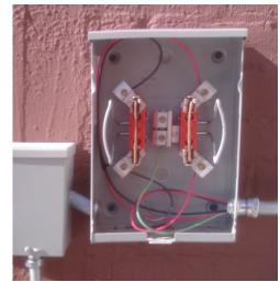
Several more calls and emails between DTE and the electrician we understood the issues and the electrician agreed to change the meter socket. What is needed is to add a fifth jaw to the meter socket to add a ground/neutral to the socket. The electrician was able to locate this part and has ordered it. Unfortunately, he then had a scheduled trip out of town for two weeks and as of the end of February, the extra part has not yet been installed.
