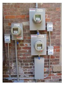
working, but we now need to convert the pulses into kilo-watt-hour data. The picture to the left shows the three utility meters used for net-metering with DTE Energy. Note the small "Customer Access Enclosure" boxes next to the meters. This is where we connect our wires to read the meter. The conduit connecting these boxes contains standard phone wire to bring the data into the store. The program is being written by volunteers Paul Haas and Dave Strenski.
