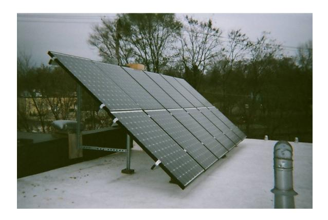
We continue to work on the design the rack for the bakery's solar panels. We have built a prototype frame and placed it on the roof to better understand how it will integrate into the "shed roof" which is on top of the building.
