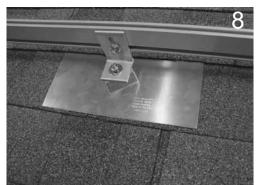
Insert EPDM Rubber Washer over Hanger Bolt Using the Rack Kit Hardware, secure the rack of your choice (see 9\*). Tighten to 16 foot pounds.
