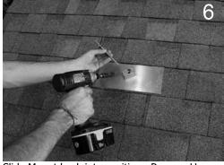
Bolt with 1 Hex Nut and 1 Sealing Washer, insert through Block into hole and drive Hanger Bolt into rafter, tightening to 13 foot Pounds.
