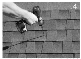
into roof and rafter, taking care to drill square ant. to the roof. Do not use Mount as a drill guide.
