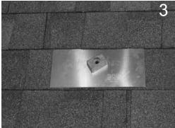
Locate, choose, and mark centers of rafters to Lift Composition roof shingle with Roofing Bar, Slide Mount into desired position. Remove any nails that conflict with getting Mount flush with front edge of shingle course. Mark center for drilling.
