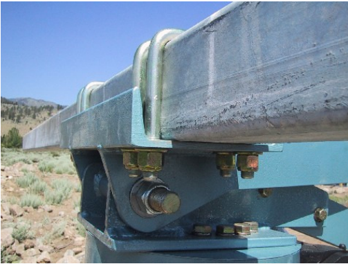
TIGHTEN NYLOCK 5/16" U-BOLT NUTS EVENLY .
