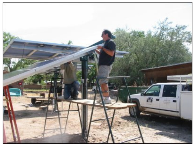
Lifting and bolting the sub-array onto the tube. Typically a 3-person job: 2 lifters, 1 bolter. Lift by the tracker rails only, not the module frames!
