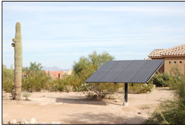
Wattsun™ AZ-225 Single Axis Tracker. 2.4 kW Residential installation.
