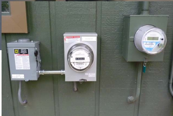
Meters and panel outside of garage
