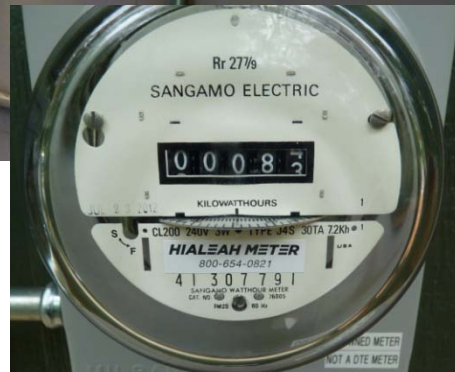
Meter monitor of KW produced Installed 2 days prior to photo
