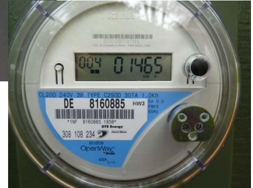
DTE Meter of KWH minus energy produced by solar
