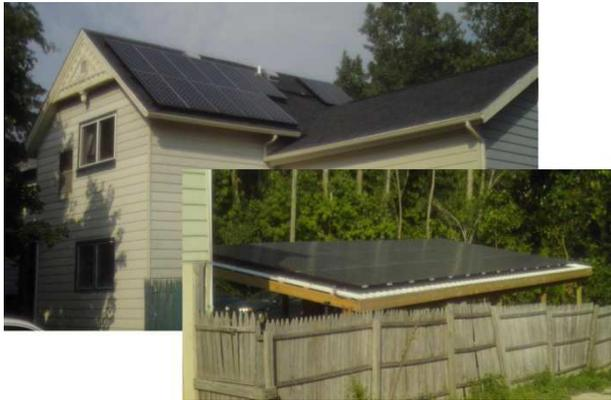
The total system cost was \$82,000 but after incentives his out of pocket cost was \$24,000 and the estimated ROI is 5 years. The system consists of 55 SunPower solar panels and Enphase micro inverters. The system was installed by Oak Electric and took about two months from start to finish.
