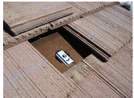
Typical standoff base installation
