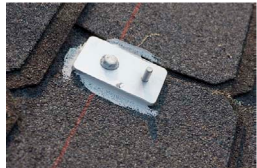
Apply sealant and secure base to rafter
