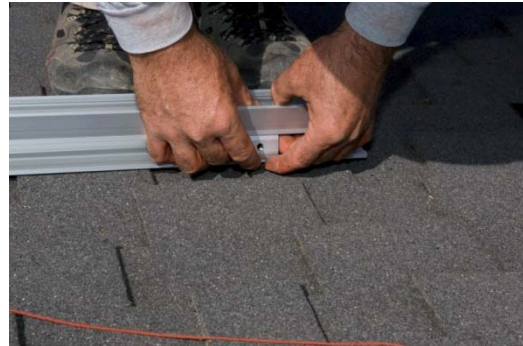
Snap in channel nut
