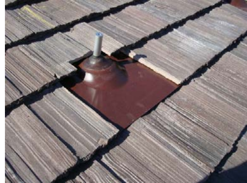
Standoff installation using Oatey flashing
