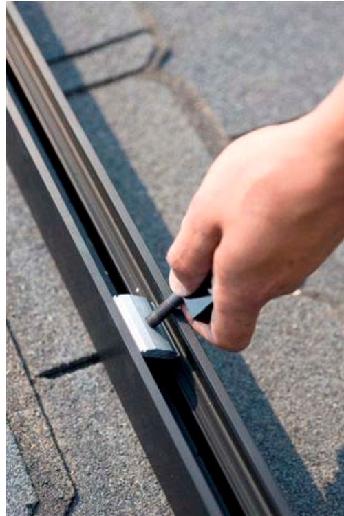
Snap module clamp assemblies into rail
