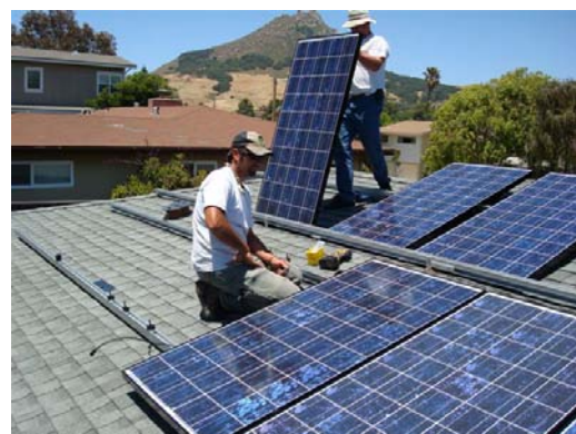
Installing modules
