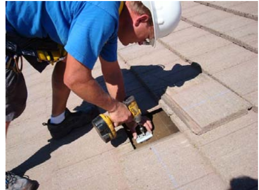
Secure standoff base to rafter
