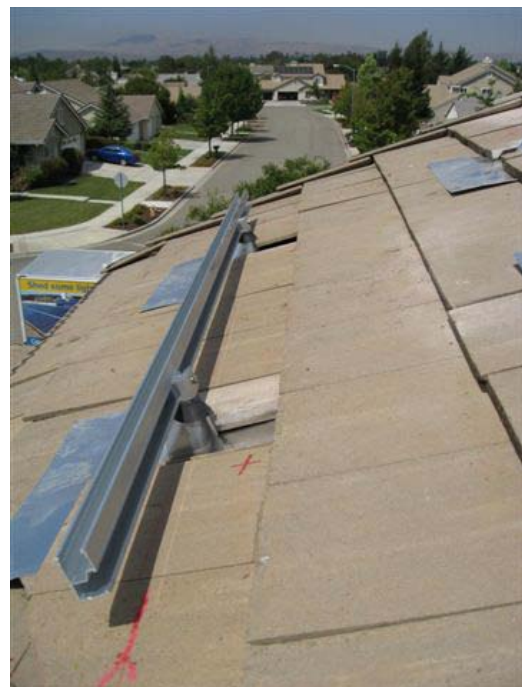
Downslope mounted rail
