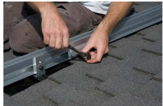
Tighten bolts on splice
