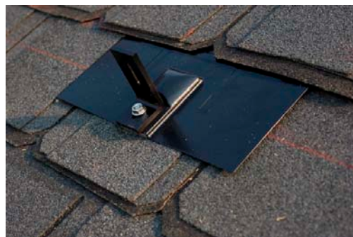
Installed L-foot assembly
