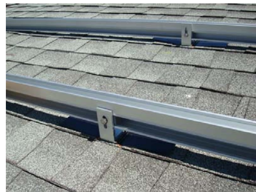
Standard rail mounting configuration
