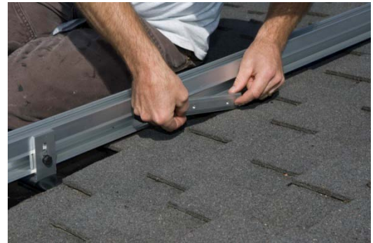
Snap in splice insert
