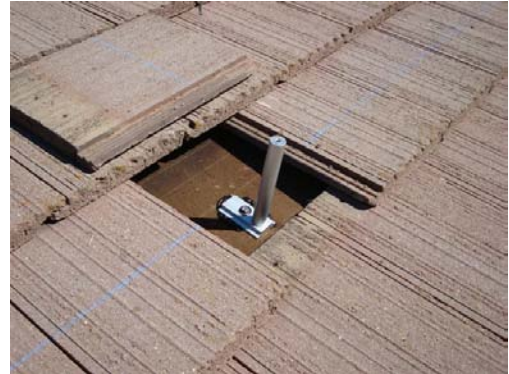
Screw standoff onto base
