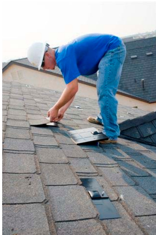
Install flashing
